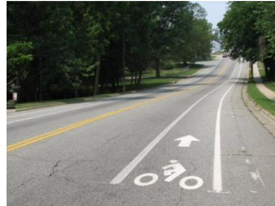
Figure 5: Bike Lane; Source: www.richmondva.wordpress.com
