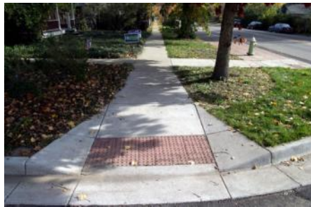
Figure 1: ADA-compliant sidewalk; Source: Pedestrian and Bicycle Information Center
