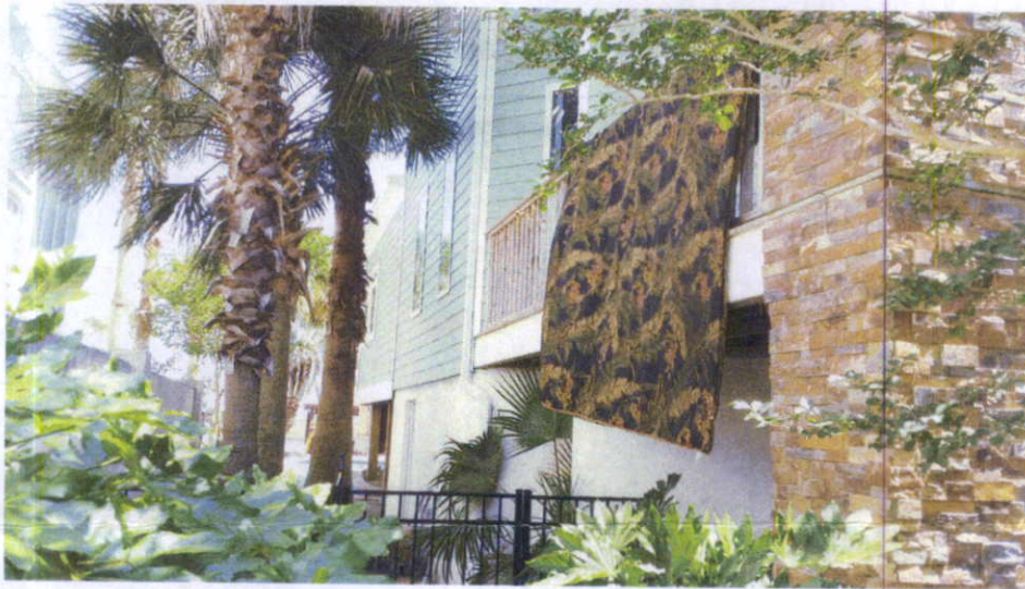
FRONT VIEW (STREET SIDE) PHOTO TAKEN 5/27/2016
