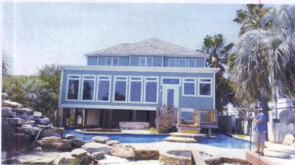
REAR VIEW (CREEK SIDE) PHOTO TAKEN 5/27/2016
