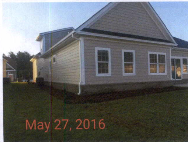
Rear Right Side HVAC
